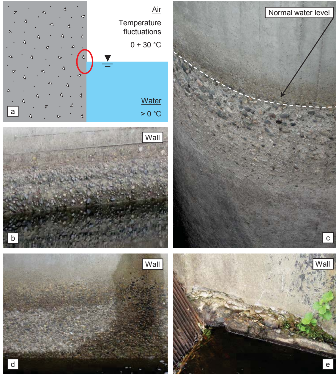
Figure 2-6. Temperature conditions at the waterline are shown in (a). Photos (b–d) show three examples of surface deterioration of concrete at the waterline of hydro power structures. Photos (b–c) are taken on the upstream side whereas photo (d) is taken on the downstream side. Photo (e) shows an example of internal damage above the waterline.
