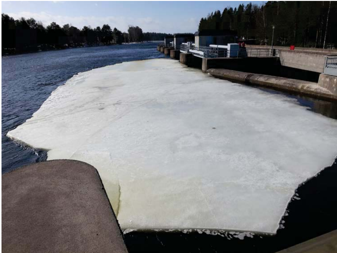
Figure 2-5. Ice floe pushing against the dam and a bridge pile.
