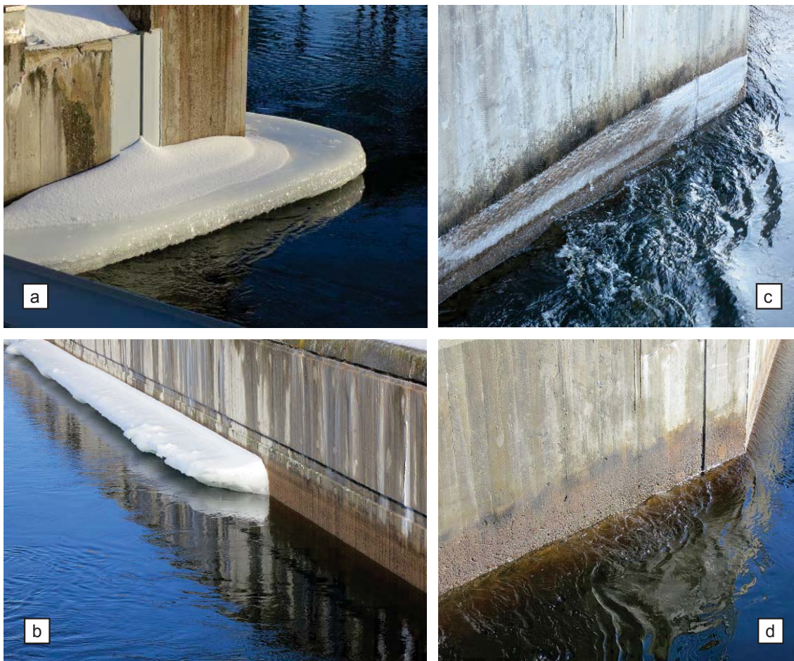
Figure 2-3. In winter, a band of ice frozen solid to the concrete surface can be seen at the waterline of hydraulic structures (a). In spring, the band of ice falls off when the air temperature rises (b). In both spring and autumn, the air temperature frequently crosses the freezing point of water. A small band of ice can therefore be seen at the waterline in the morning (c) while it has been melted away in the evening (d).
