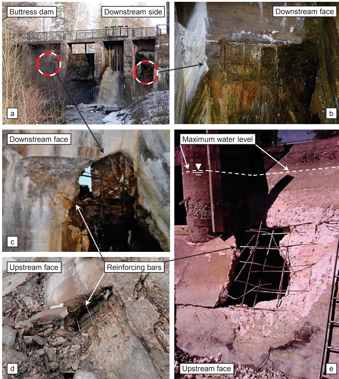
Figure 2-11. A severely damaged buttress dam (a). Concrete cover missing in some places in the vicinity of water leakage through cracks on the downstream face (b). A hole appeared in the flat slab in another place and water escaped flushing away loose pieces of concrete (c–e). Only the reinforcing steel was left. Photos provided by Fortum AB.
